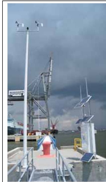
The new real-time wind and current station.
